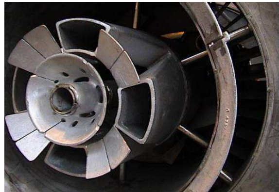
Fig. 6 - Standard TEA-C Low-NOx Burner
