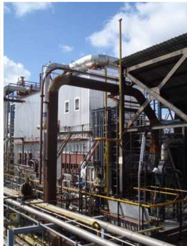
Fig. 4 – Pneumatic feeding components
